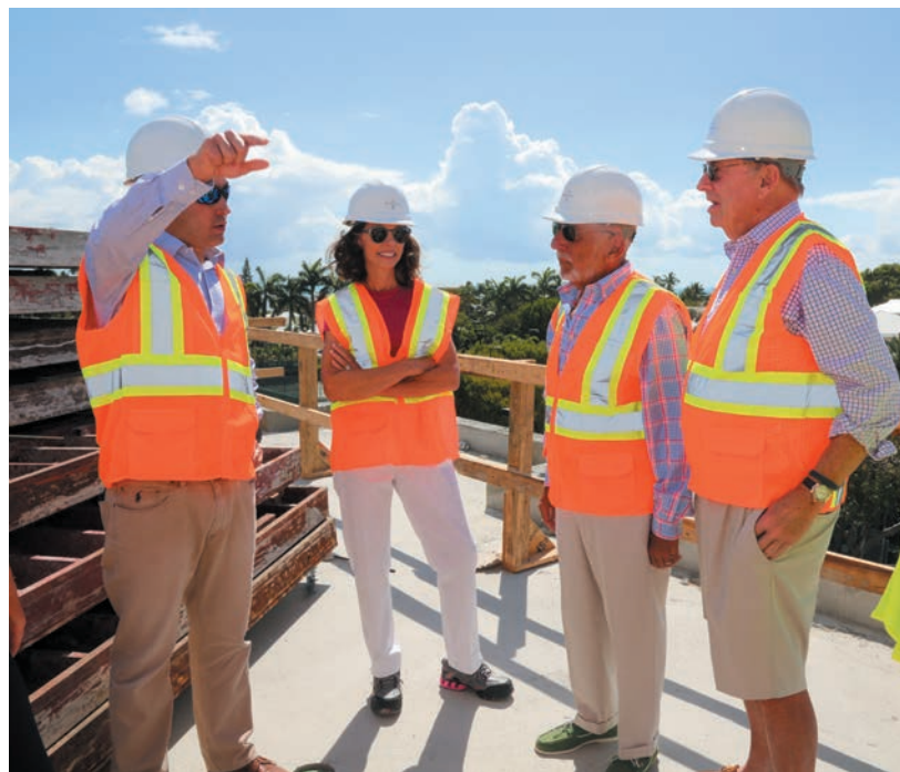
Eric Soulavay shares details on the construction process with Board Members Teresa Holmes, Bob Schmetterer and Don Waite.
